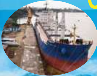
Jetty Service and Berthing Facility
